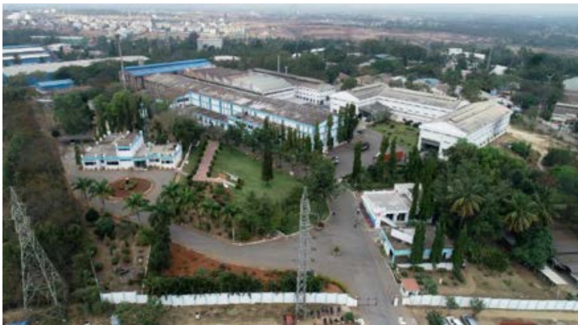
Ariel view of manufacturing plant located at Mysore, HO
